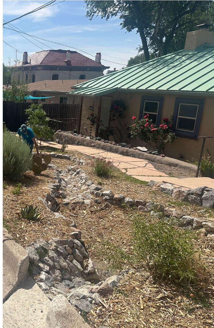
A green stormwater infrastructure (GSI) feature with curb cut, bioswale and basins in Silver City constructed by Asher Gelbart, Green Energy Now, that will harvest rainwater to irrigate the landscape and reduce flooding in streets during storm events.
