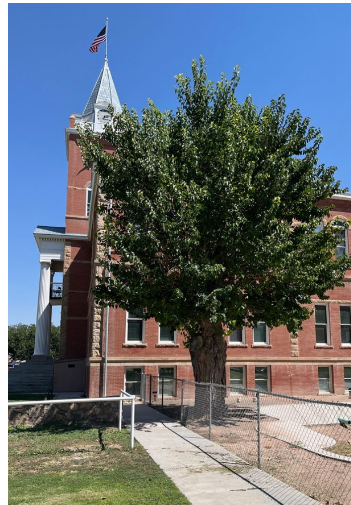
The Luna County Courthouse is on the National Register of Historic Places. The landscape requires a tree maintenance, removal and succession planting plan to maintain this historic landmark's beautiful presence in Deming.
