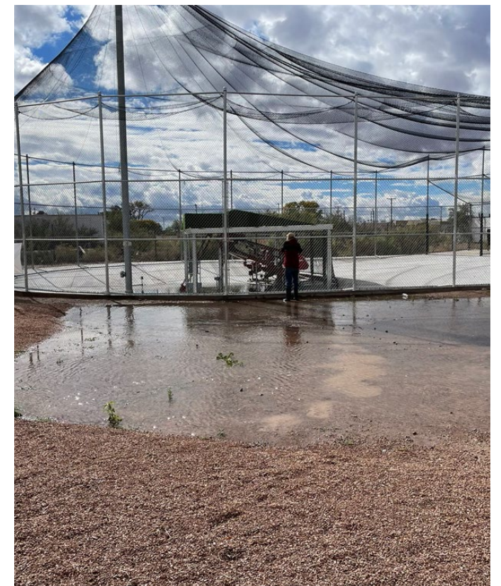
Flooding at Inclusive Park and the Starmax batting cage. GSI practices can re-purpose stormwater to irrigate plants, creating a more vibrant and beautiful city while helping to address flooding problems.
