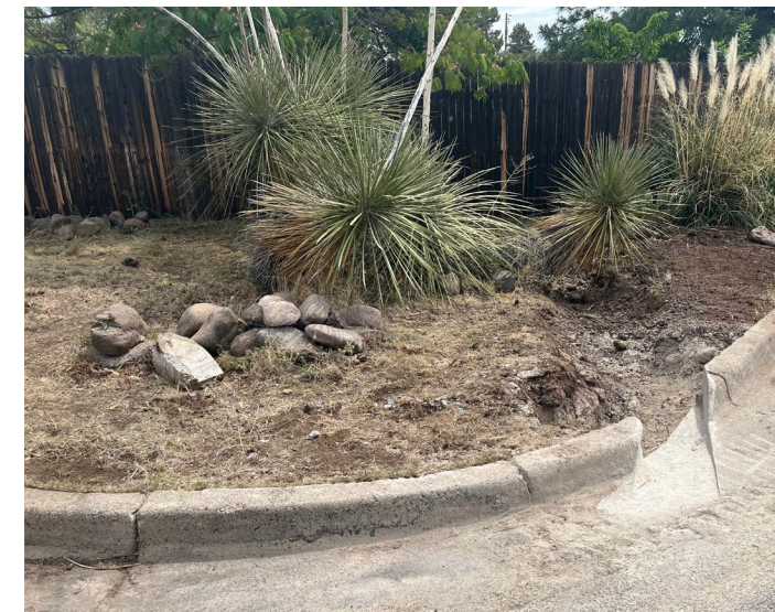
Photos above and below show examples of green stormwater infrastructure in Silver City neighborhoods. Curb cuts and water harvesting basins were installed by Van Clothier with Stream Dynamics.
