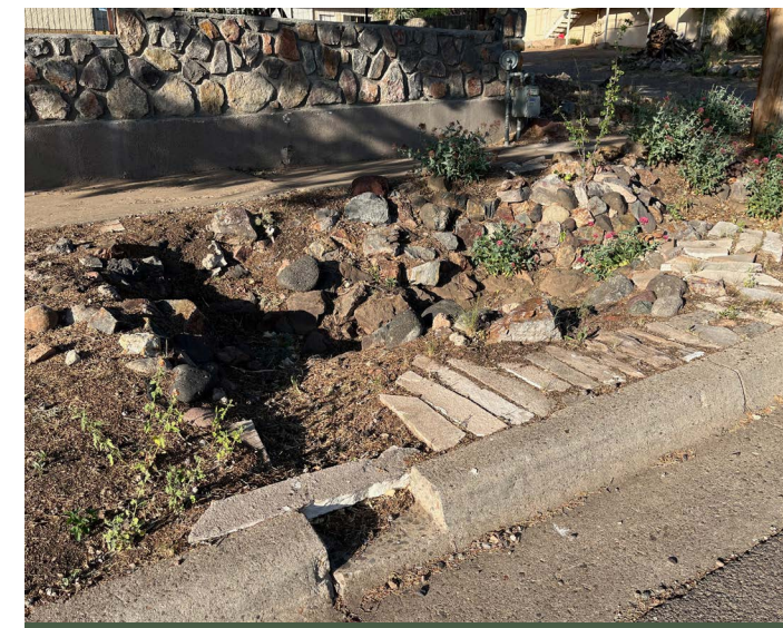
Photos above and below show examples of green stormwater infrastructure in Silver City neighborhoods. Curb cuts and water harvesting basins were installed by Van Clothier with Stream Dynamics.
