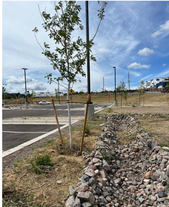
New tree plantings at the Silver City Recreation Center, supported by GSI features that capture parking lot runoff and reduce the use of drinking water for irrigation.
