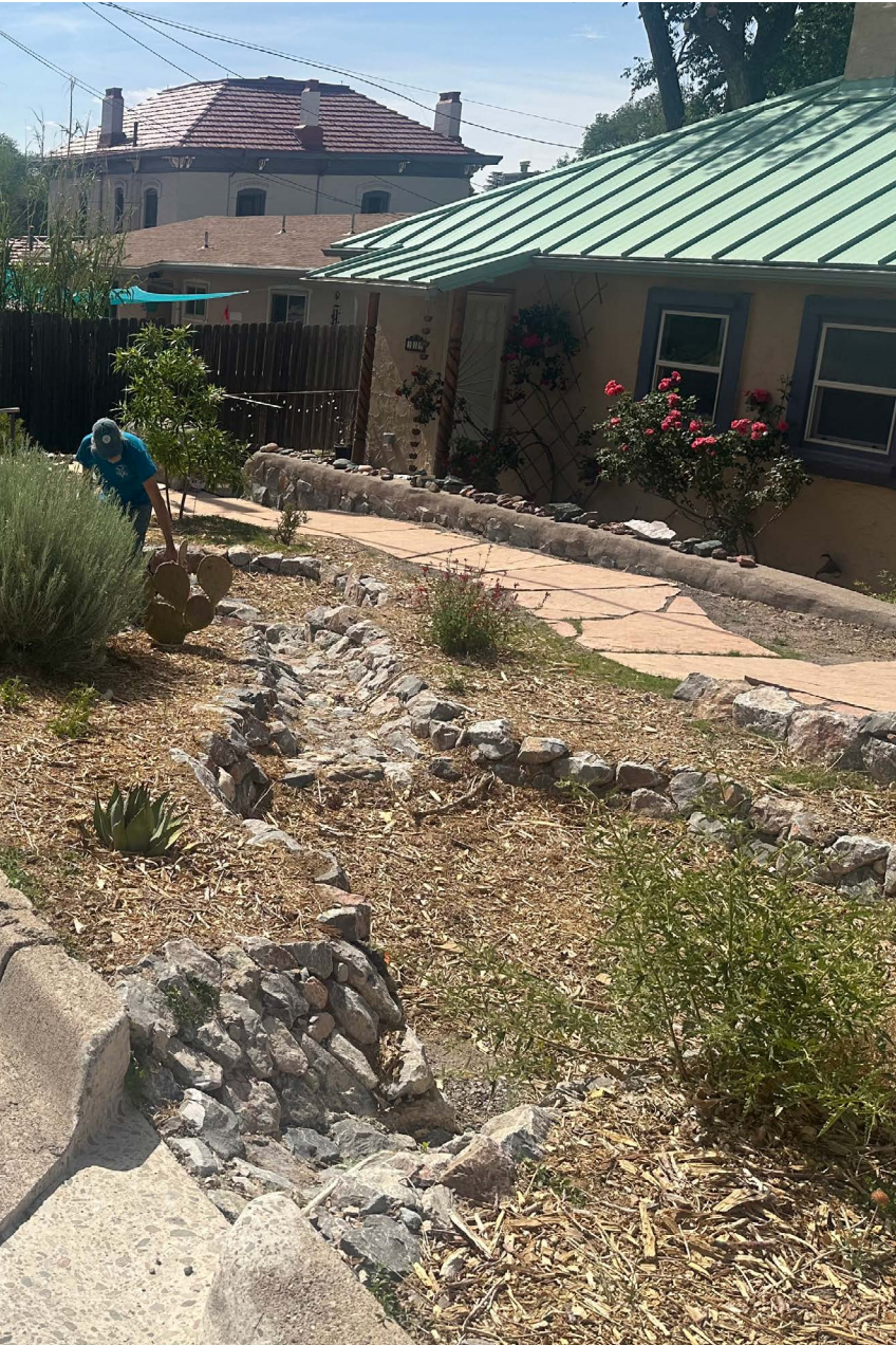
Curb cut, bioswale and basin complex in Silver City constructed by Asher Gelbart, Green Energy Now, that will allow stormwater to irrigate the landscape and reduce flooding in streets during storm events.
