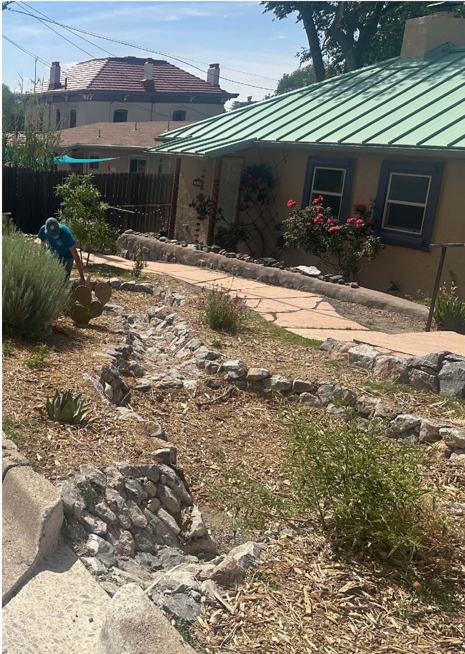
Curb cut, bioswale and basin complex in Silver City constructed by Asher Gelbart, Green Energy Now, that will allow stormwater to irrigate the landscape and reduce flooding in streets during storm events.
